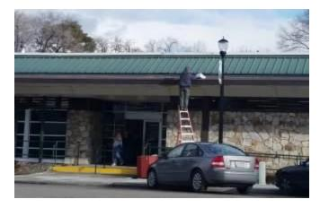
able to absorb the water runoff. If not, we may need to install an additional gutter downspout that angles back to the building and route the outlet to the street. A gutter there would be more disruptive to the visual line and appeal of the building architecture than the rain chain, so we're hoping the chain will work.
