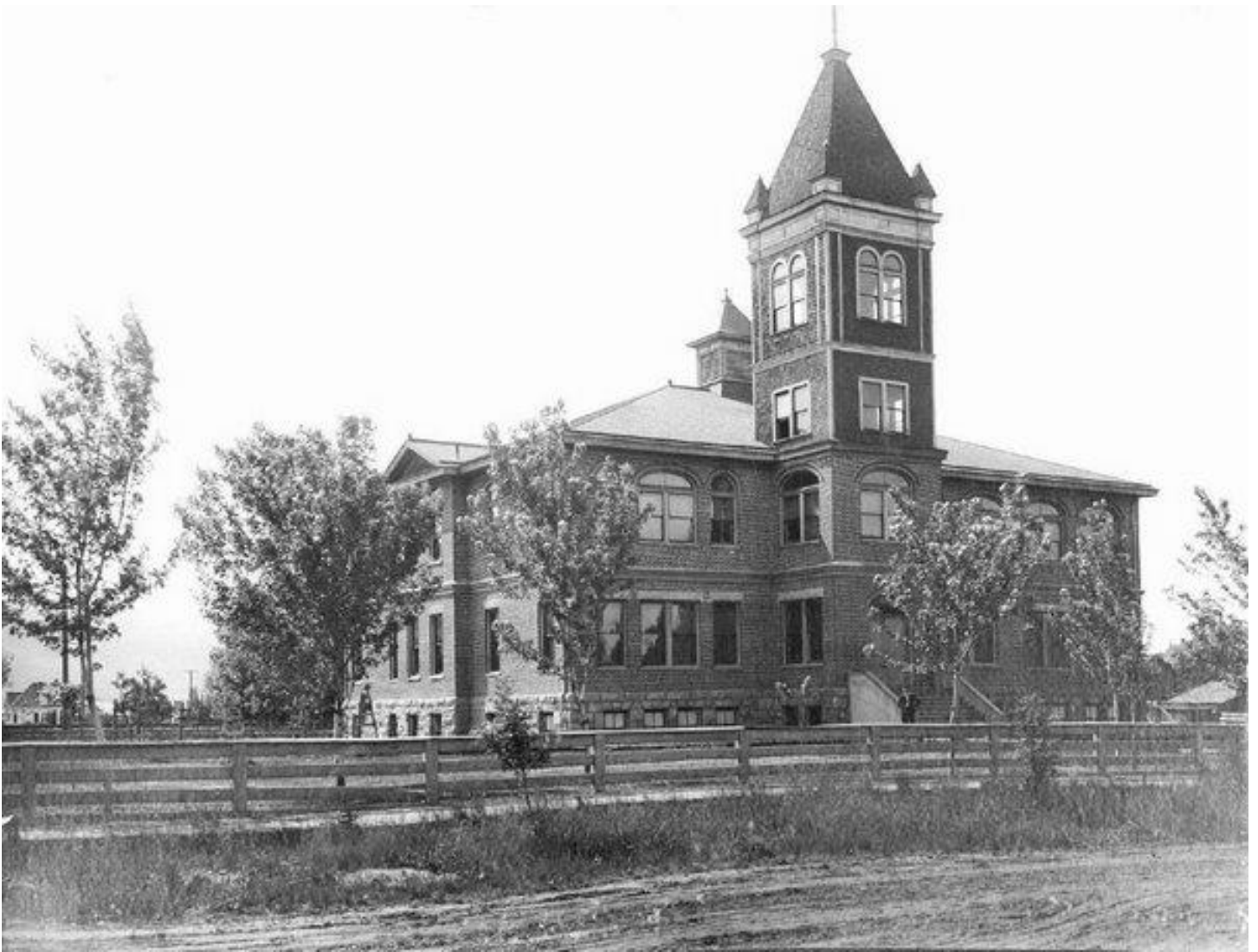
Tiedemann Elementary School, constructed 1901, just north of the Union Pacific Railroad tracks.
