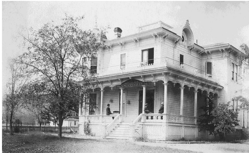
Faull House, East and North Sides
